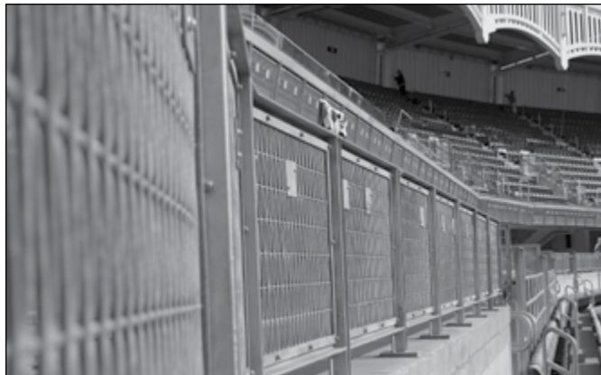
Infills of 3"x1" Rectangular Opening Flat Top Plain Weave HD Galvanized
