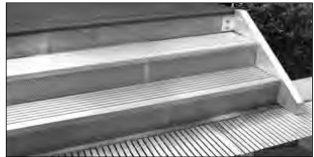
Unique stairway has SAFE-T-GRID® stairs and perforated risers
