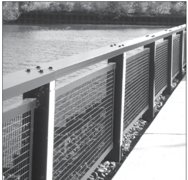
Infills fabricated of Sq. Opening Wire Mesh - 1-1/2" Mesh, .135 Wire Diameter
