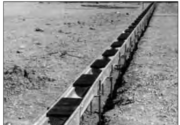
Installation process of the presloped trench drain system
