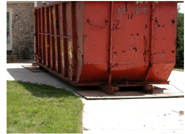
Figure 11 Large weights can crack a slab
