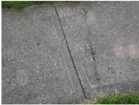
Figure 4 A crack next to a too-shallow joint
