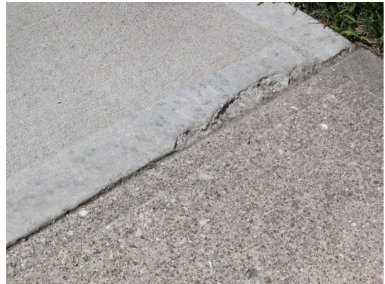
Figure 7 Expansion joint between these slabs would have prevented chipping
