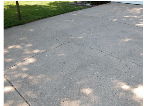
Figure 5 Driveway cracks where joints should have been placed
