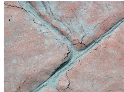
Figure 14 Crusting cracks caused by premature surface drying
