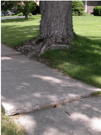
Figure 8 Tree roots lifted and cracked this sidewalk
