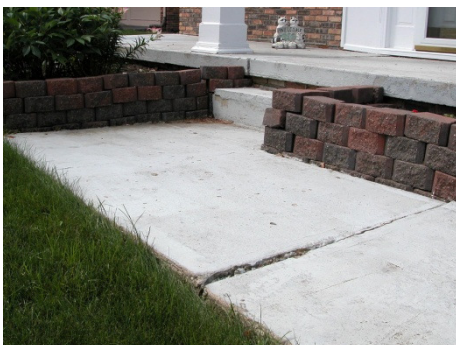
Figure 10 Sidewalk and step settled back toward the house. Note that the step has been capped to compensate
