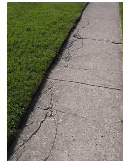
Figure 12 A heavy truck drove over this sidewalk, cracking the edge
