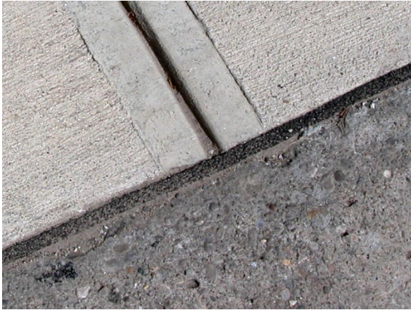
Figure 6 Foam expansion joint separating driveway and curb
