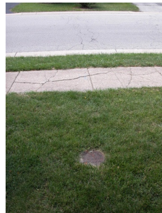
Figure 9 Note the cracks in the sidewalk and street over this poorly compacted water line trench
