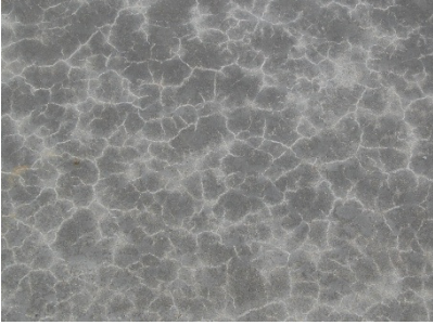
Figure 13 Crazing cracks caused by premature drying
