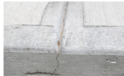
Figure 3 A successful crack control joint
