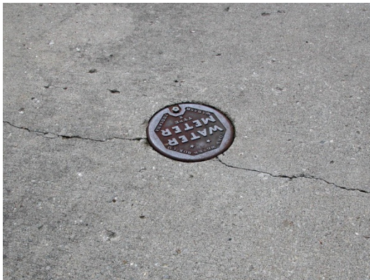
Figure 2 Shrinkage crack at slab penetration
