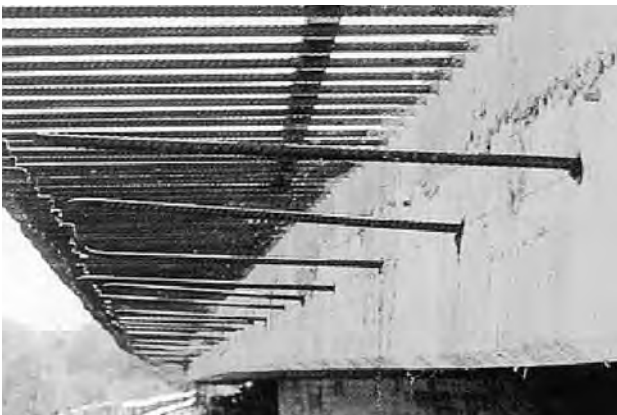
Post-installed reinforcing for widening of a bridge deck
