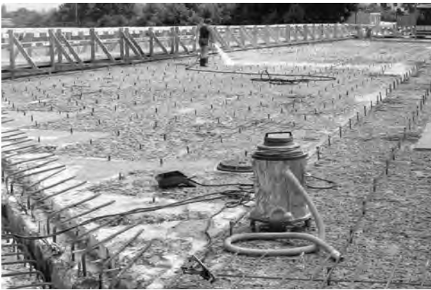
Dowels placed in preparation for a new structural topping slab
