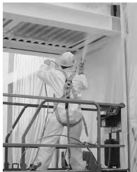
Typical Hilti Fire Protection Steel Spray application
